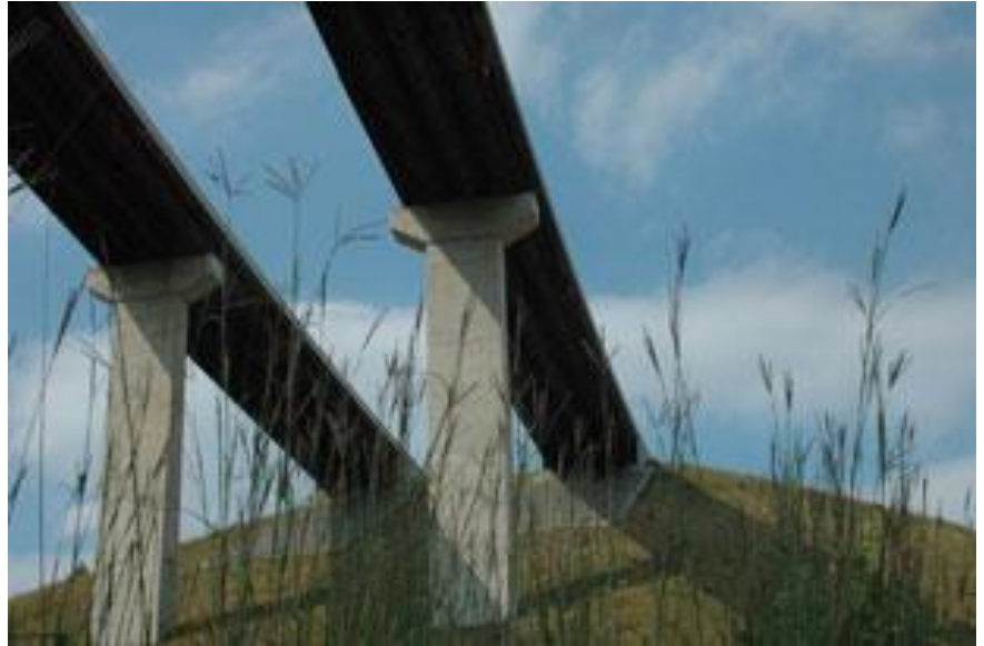
Rubles Run Bridge, Mon-Fayette Expressway (WV 43)
