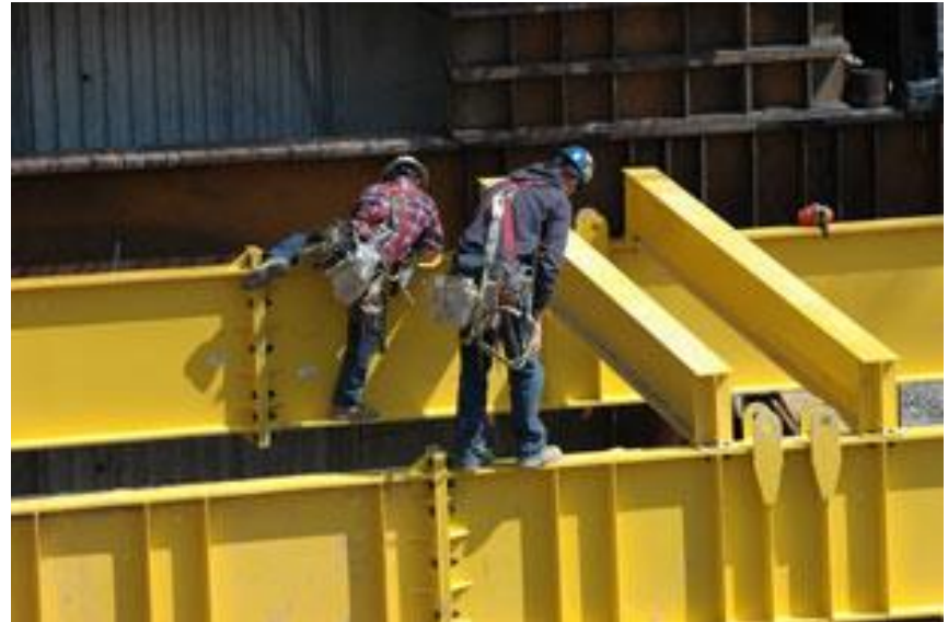
I-64 Kanawha River Bridge Oct 2008 Photos courtesy of Ahmed Mongi
