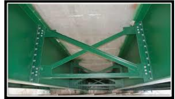
Bridge Painting, WV Turnpike
