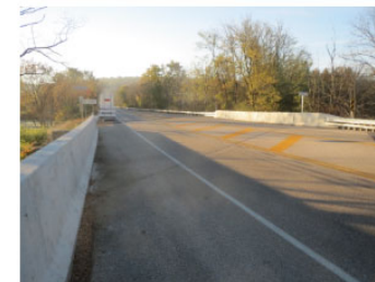
In-service bridge using modular steel superstructure elements and deck-level UHPC connections - Photo Credit: FHWA
